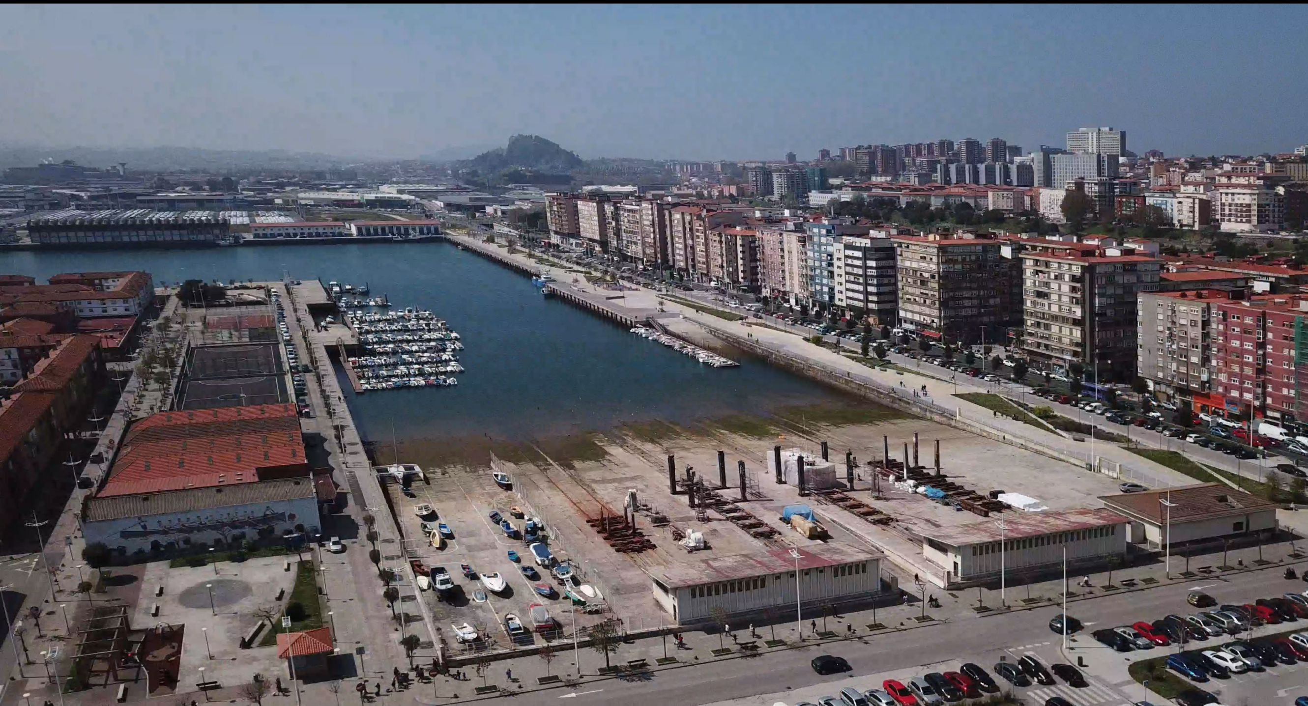
On both sides of the boat-repair dock, we can see the Castilla waterfront promenade (right) and the pedestrian street that goes along Barrio Sotileza (left). Both great existing features.
