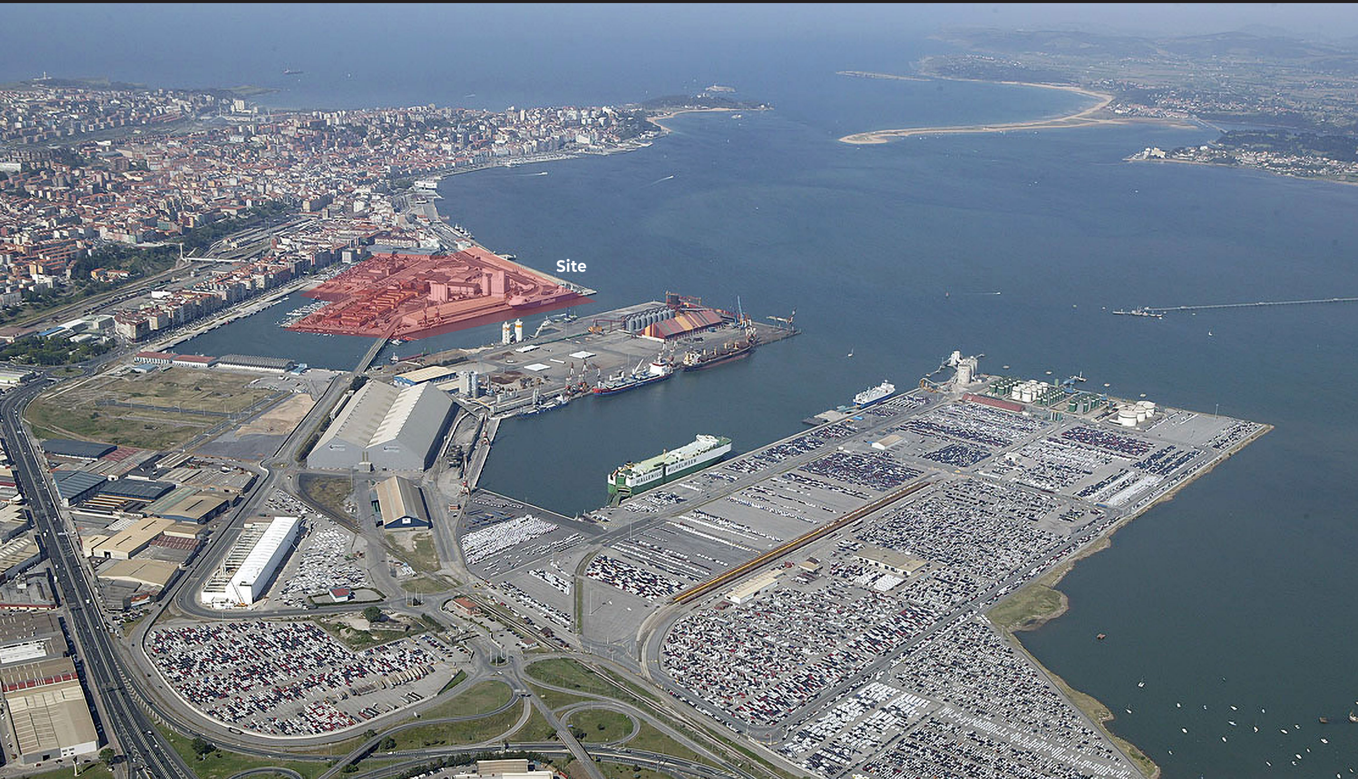
This aerial picture shows the expanded docks and how Barrio Pesquero is the meeting point between them and the city. All the flat land is artificial landfill, including the site and Castilla district. The port activity has been gradually leaving the city, and moving into the expanded docks.
