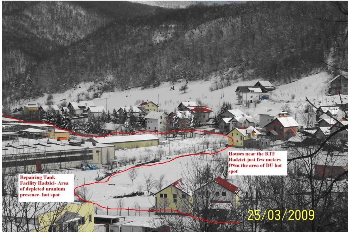
Figure 1. Repairing tank facility and settlement nearness (A.Miholjic, 2009)
