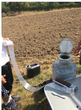
(a) Plastic hosepipe cut at a length so that it reaches from the bottom of the measured borehole depth to the top of the borehole opening.
