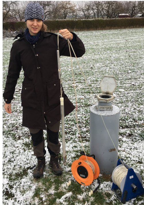
(b) Point injection device held in a way that prevents the liquid from pouring out. (Photo: Nikolai Fahrmeier)
