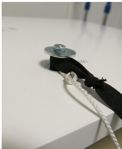
Figure 3.26 Close up of the bolt, the nut and the washer.
