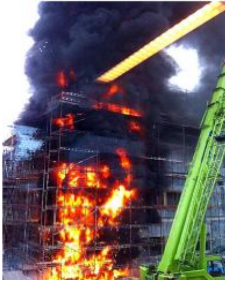
Figure 9 Façade fire in Karlstad, 2013 [24]
