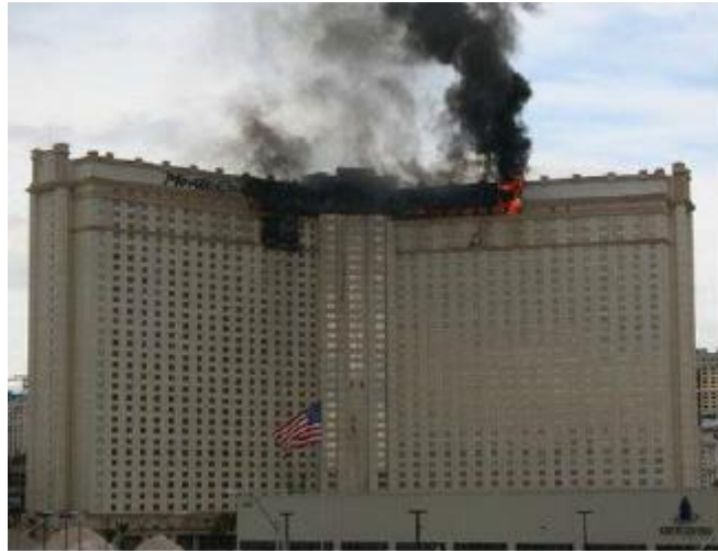
Figure 5 MGM MONTECARLO façade fire, 2008 [17]
