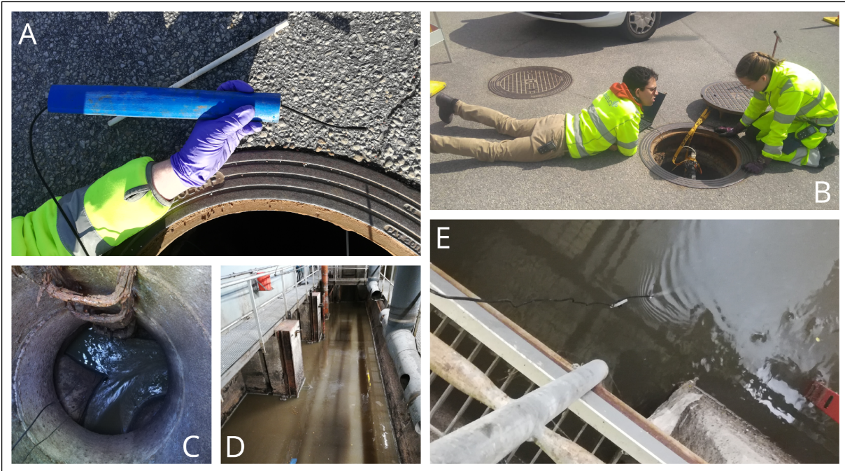
Figure 3.11. A. Protection of the sensor's cable against rat's bites; B. Data collection in the well SNB 2417 using the computer and the logger; C. Intersection of two flows in the well SNB 2417; D. Inflow basin at Rosendal PS; E. Sensor at Turbinen PS with the metal weight.
