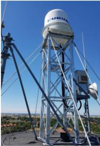
Figure 11 The weather radar station in Dalby in 2018 (South et al., 2019).
