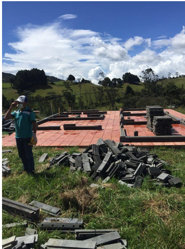
Figure 20: Preparation before construction on a concrete slab (Conceptos Plasticos n.d.)
