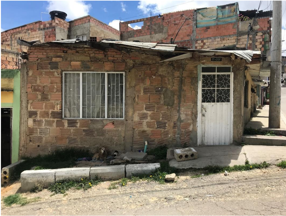
Figure 17: Masonry house with commonly used windows, door and roof (Photo by authors)
