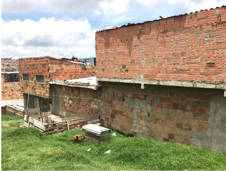
Figure 15: Non-reinforced masonry in Usme, Bogotá (Photo by authors)
