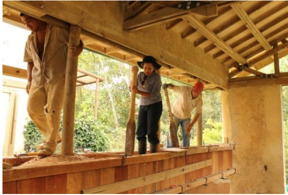
Figure 7: Construction of a wall of Tapia pisada (Flickr, 2011)
