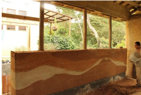
Figure 8: Finished wall of Tapia Pisada (Flickr, 2011)
