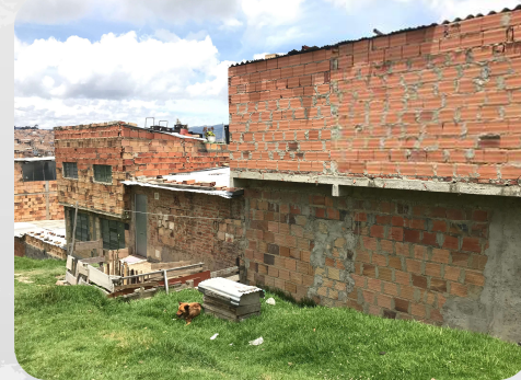
Figure 3. Inadequate masonry houses in Usme.
