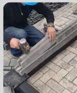
Figure 6. Method of mounting plastic bricks.
