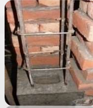
Figure 4. Column ready for casting.
