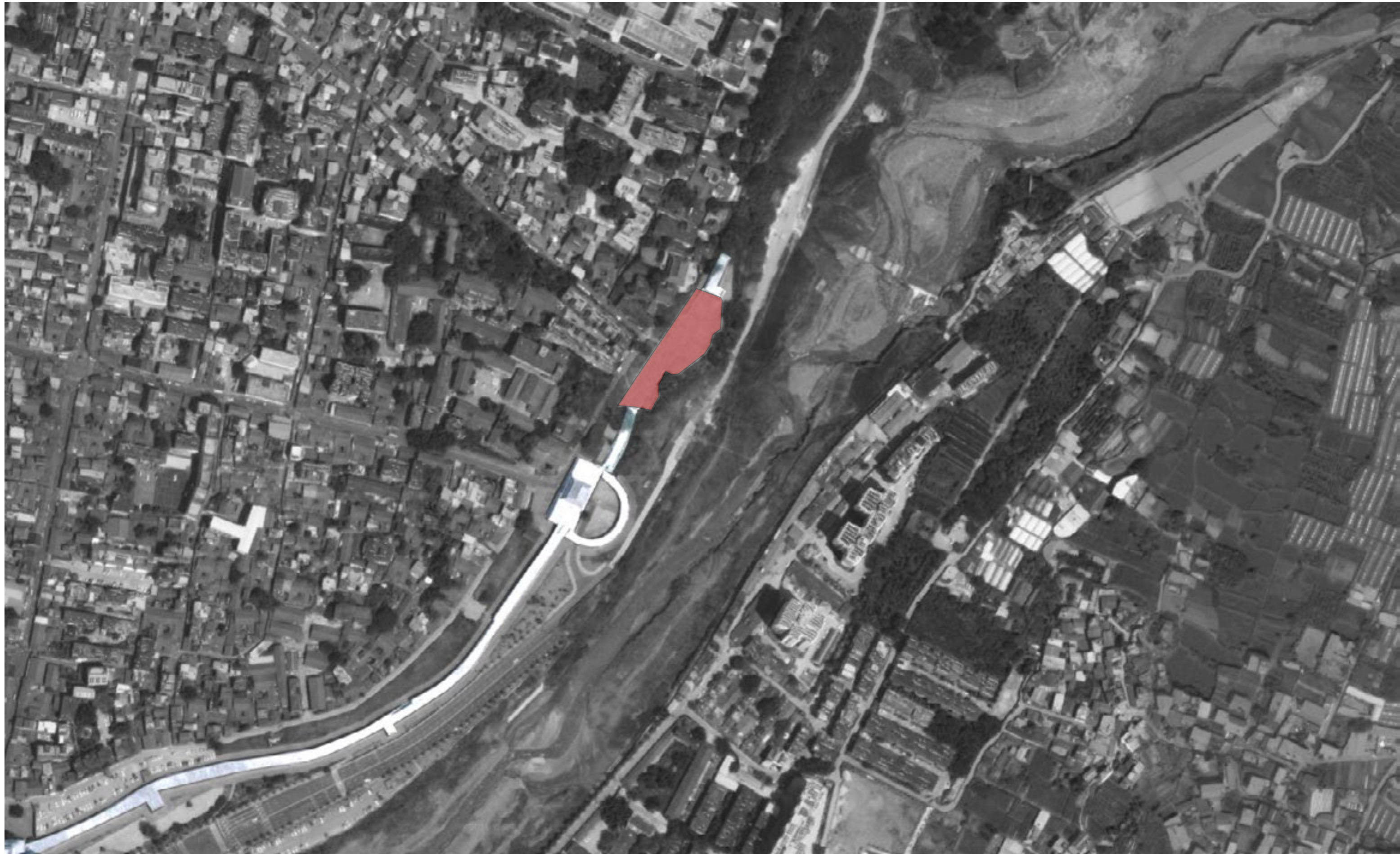
One damaged part of the relic wall
