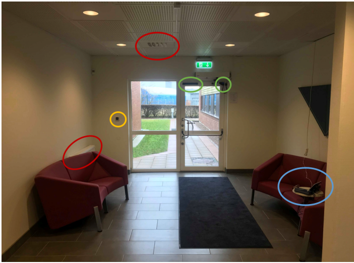
Figure 4.1: The setup for the field study is shown. The Blue circle encircles the temperature measurement position, the yellow circle is the activation button, the red circles show the ventilation, and the radiator and the green circles encircle the two sensors. The leftmost green circle is the old safety sensor, and the rightmost is the new TOFSwing.
