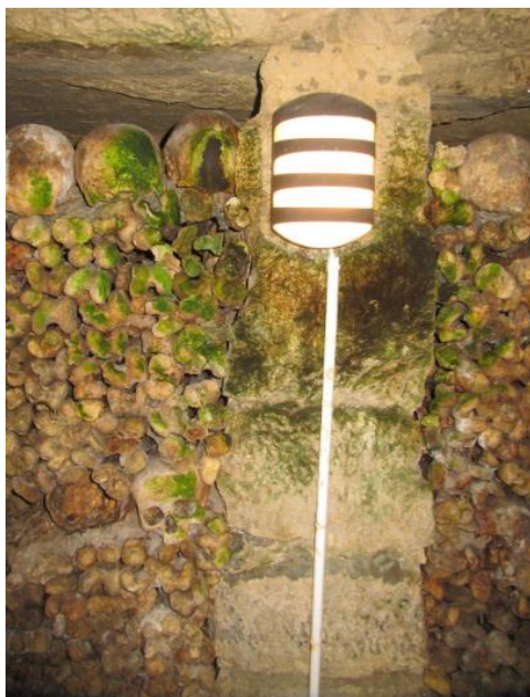
Figure 20: Development of invasive species because of the lighting system in the Catacombs Museum (Source: http://paris-bise-art.blogspot.com/2017/08/lagonie-des-catacombes.html )
