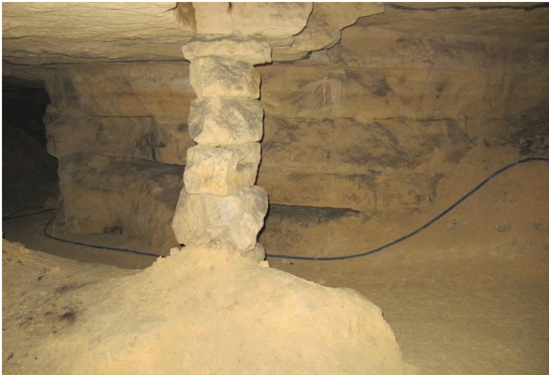
At the time the quarries were used for exploitation, miners were creating column with stacks of stones between floor and ceiling in areas where a lot of mineral were extracted. This technique is called “piliers à bras” (Picture credits: Gilles Thomas)
