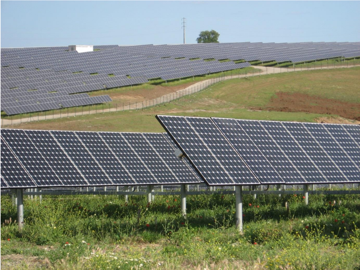
Figure 4: 11 MW grid-connected Serpa Solar Park, Portugal. (Source: Ceinturion,2006. Licensed under CC BY-SA 3.0 license via Wikimedia Commons.)
