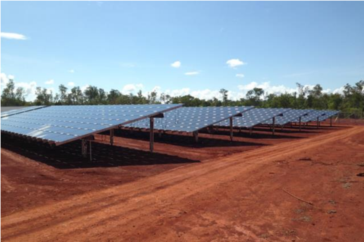
Figure 3: 6.7MW off-grid Weipa solar plant, Australia. (Source: Australian Renewable Energy Agency (ARENA), 2014. Public domain image.)
