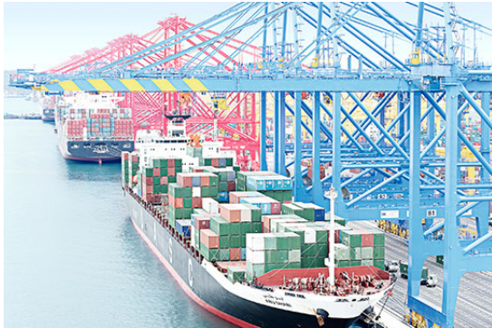
Figure 1: STS cranes loading containers onto freight ships
