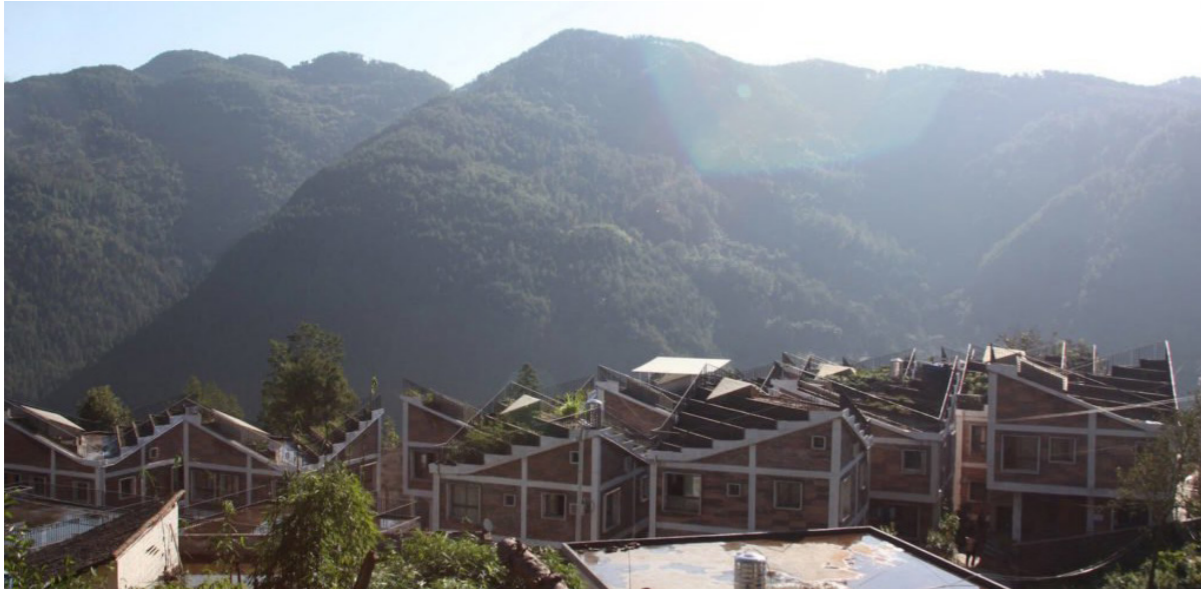
HOUSING IN JINTAI VILLAGE BY RUF
