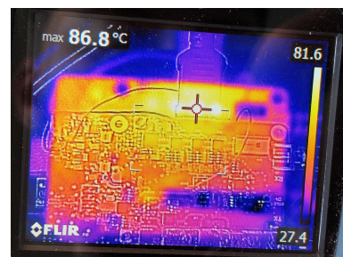
Figure 7.11: Thermal Image of the RX LNAs
