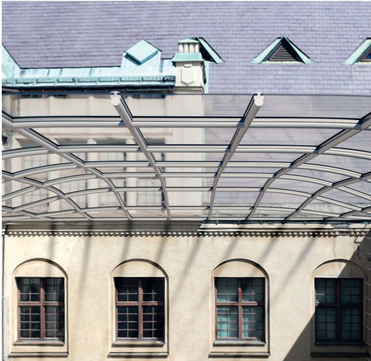
Cut through of the glass roof in Linnanpiha
