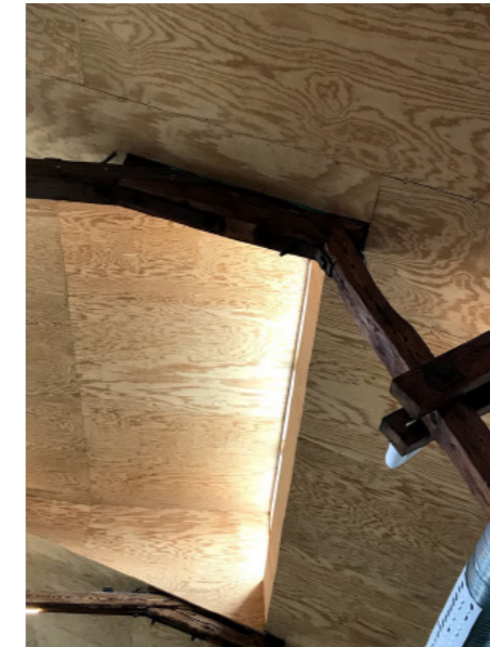
The ceiling has been fitted with a plywood cladding ←
