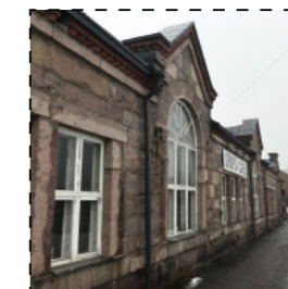
Closed monolithic facades towards the public path
