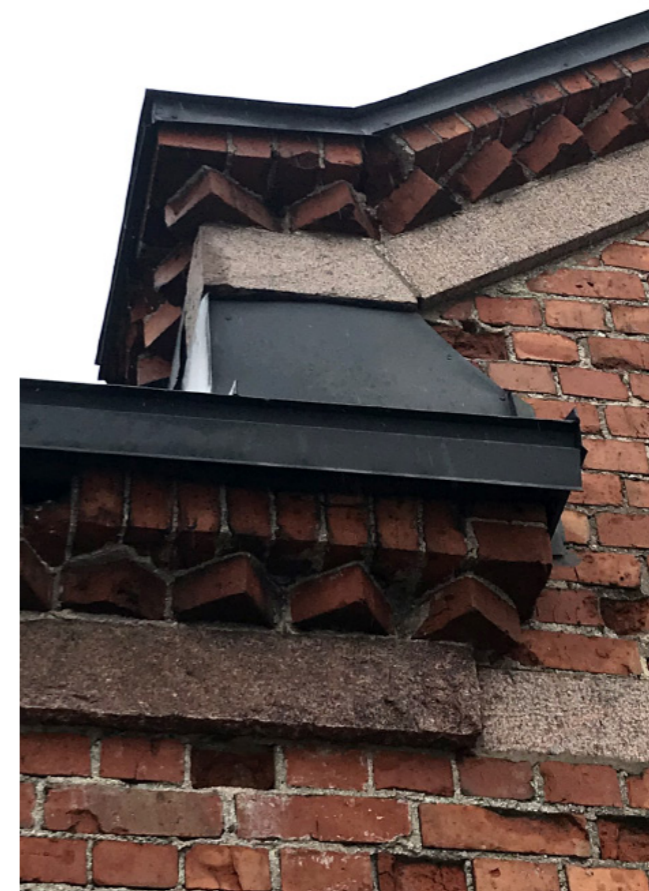
↑ Brick detail, east facade
