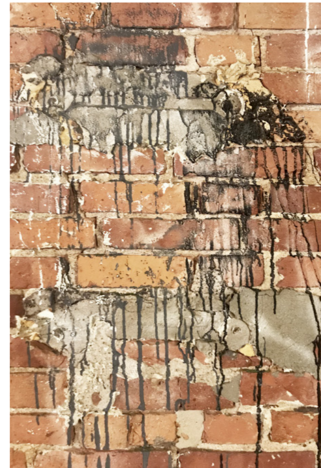
↑ Interior brick facade
