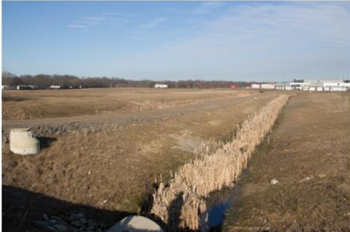
Figure 4-6: Location 2, two-stage ditch
