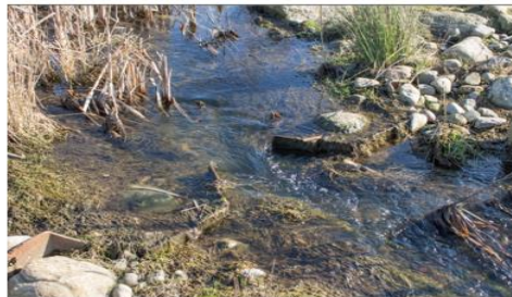
Figure 4-5: Outlet of the pond with a control structure
