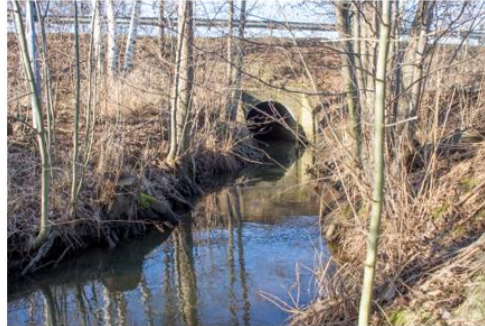
Figure 4-7: Location 3, Reshaped ditches
