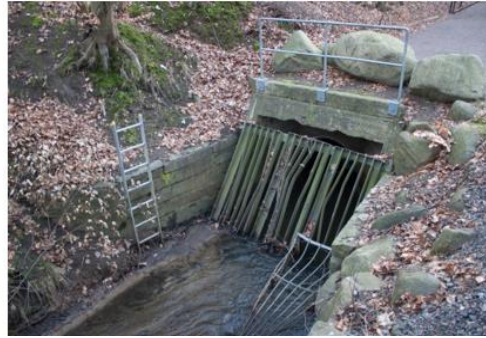
Figure 4-11: Beginning of the culvert section in the Ramlösa
