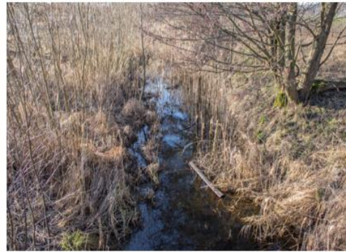
Figure 4-9: Location 2, two-stage ditch
