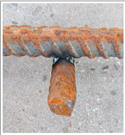
(d) Picture showing welded connection between rebars.
