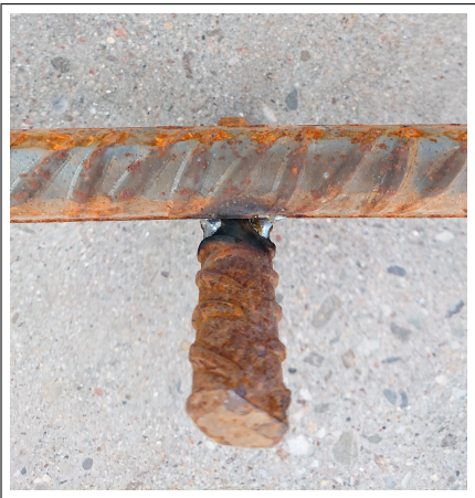
(c) Picture showing welded connection between rebars.
