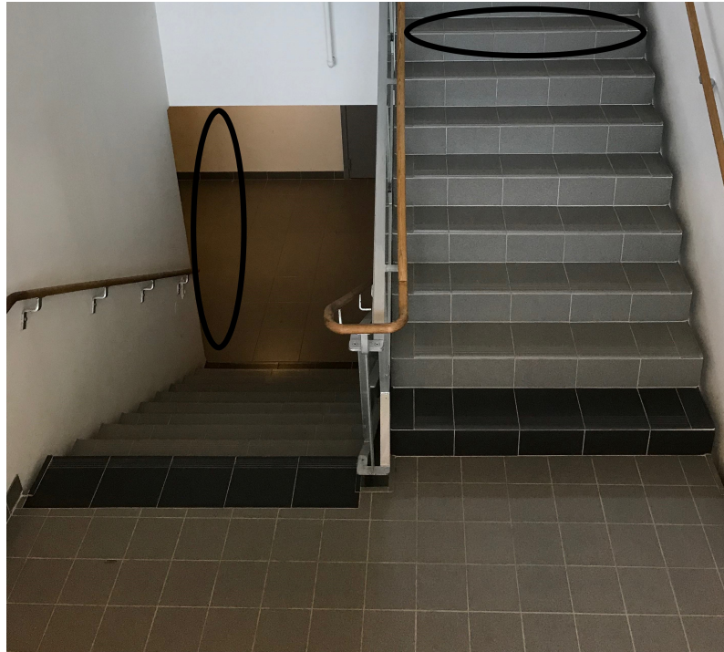
Figure 2.2: A FOV showing a stairwell. Entry/exit zones are shown with ellipses.
