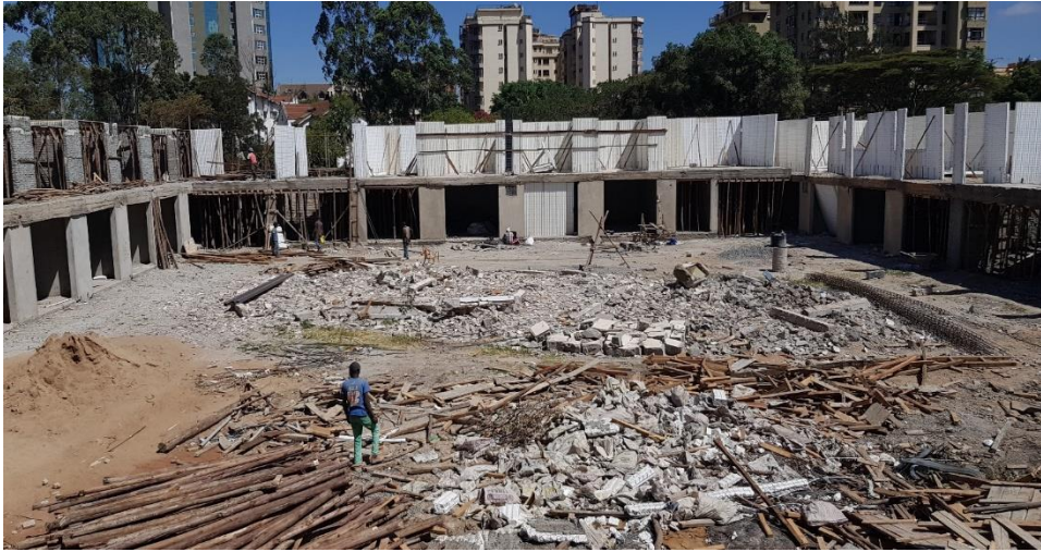
Picture 2: Hurlingham Shopping center construction site
