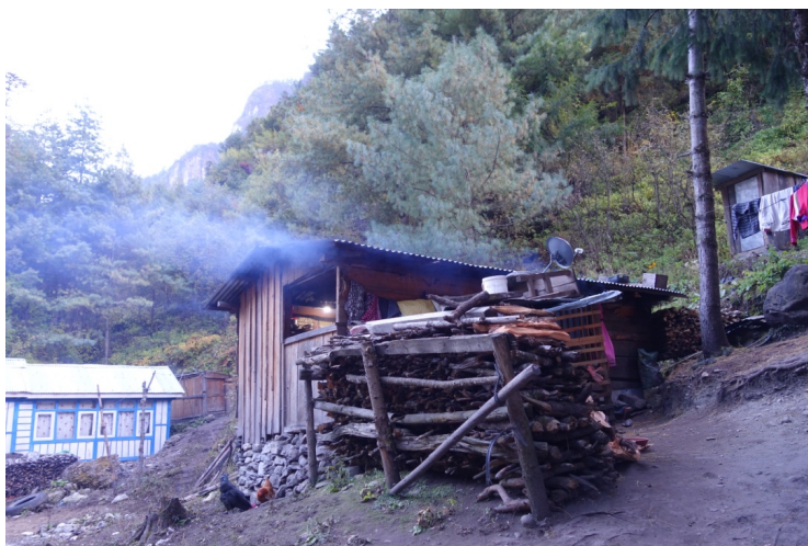
Figure 37: Stove generated smoke exiting a kitchen through an opened window and gaps between the walls and roof.
