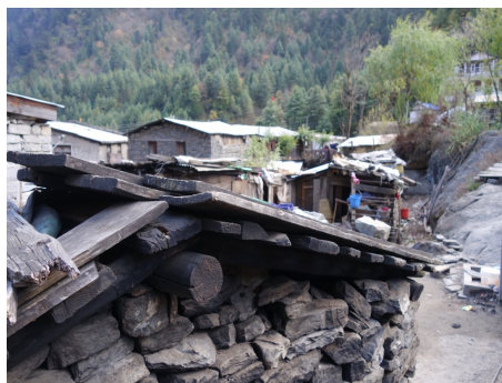
(a) Roof of wooden planks.
