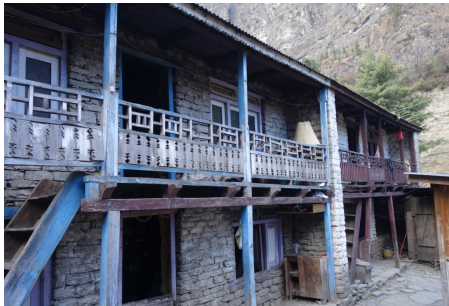
(a) Type of house construction referred to as typical Chame house.
