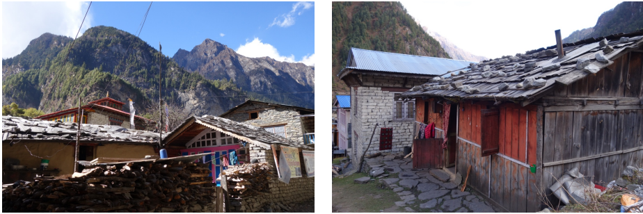
(a) Mud-brick bonded walls.
