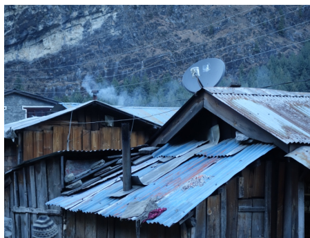
(b) Roof of corrugated steel
