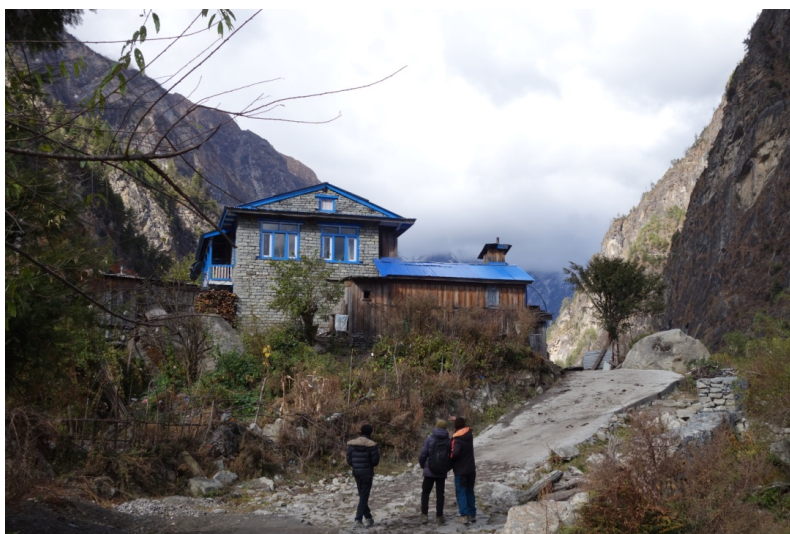
Figure 15: Example of a separate kitchen built in wood adjacent to the residential unit.
