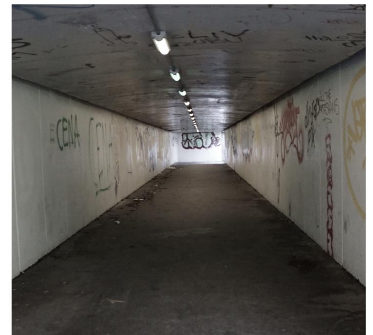
Pedestrian underpass on Frederikssundsvej. Source: Potoczniak, 2019
