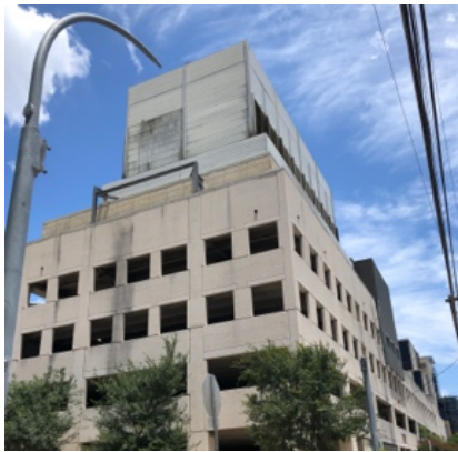
Figure 4-3: Paul Robbins District Cooling plant (DCP-1)
