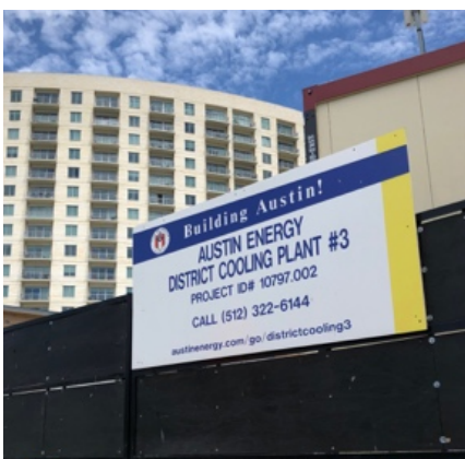
Figure 4-5: Austin Energy DCP-3
