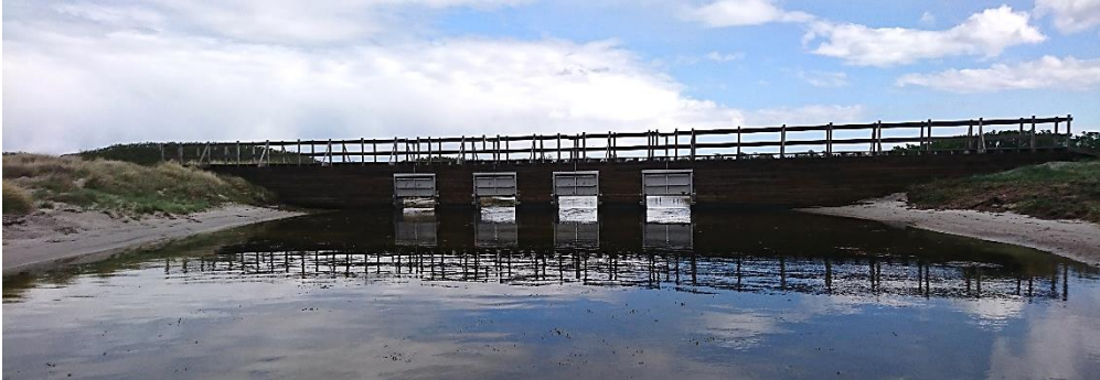
Figure 6. The sluice gate on the inlet. Photo by: Shuwei Wang.
