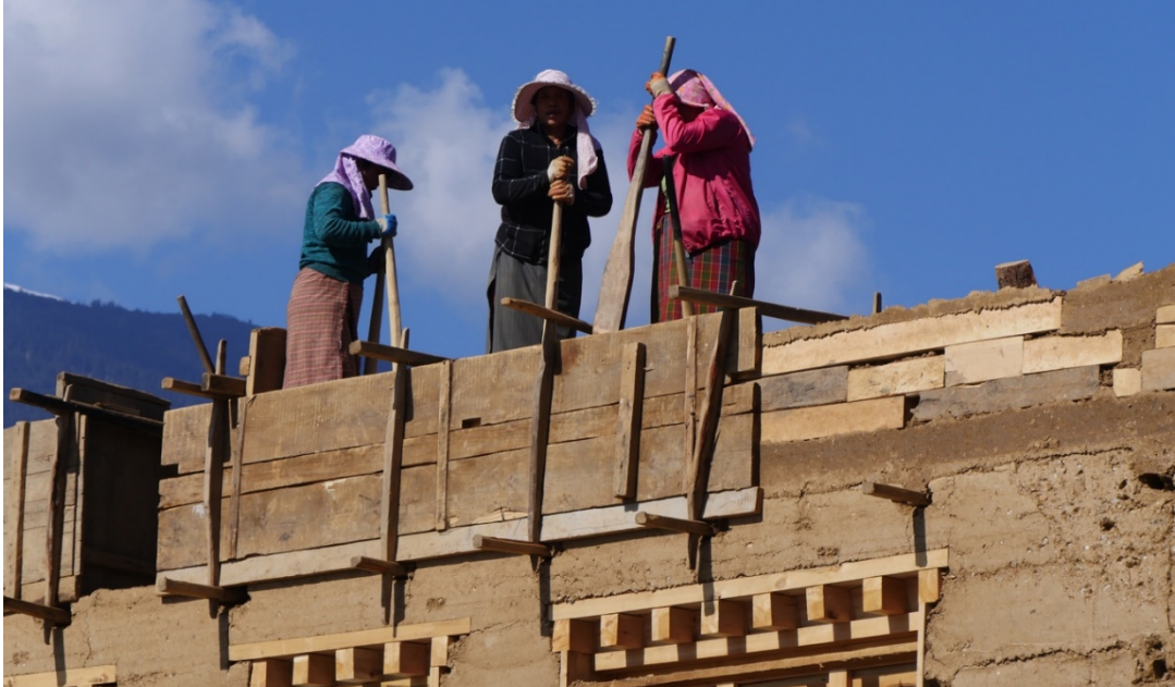
Figure 10: Three women working on a rammed earth building
