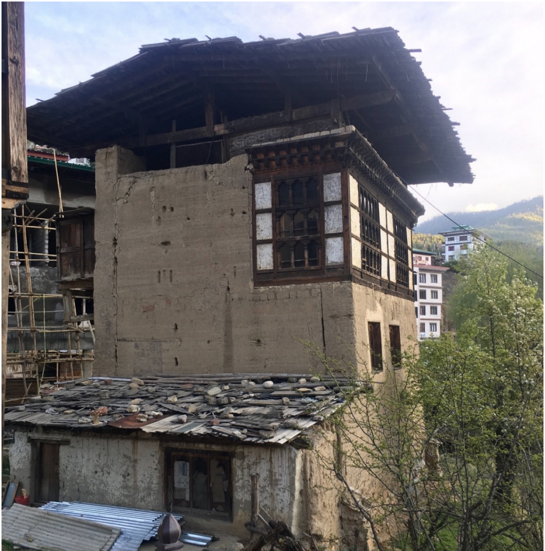
Figure 5: Typical Rammed Earth Dwelling, with on the second floor a rabsel with earth infills [12].
