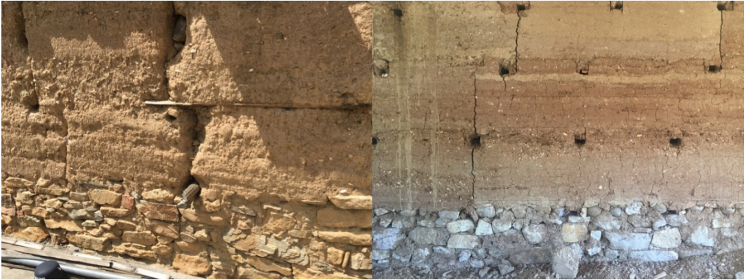
Figure 6: Rammed earth wall on traditional(left) and modern(right) plinth
