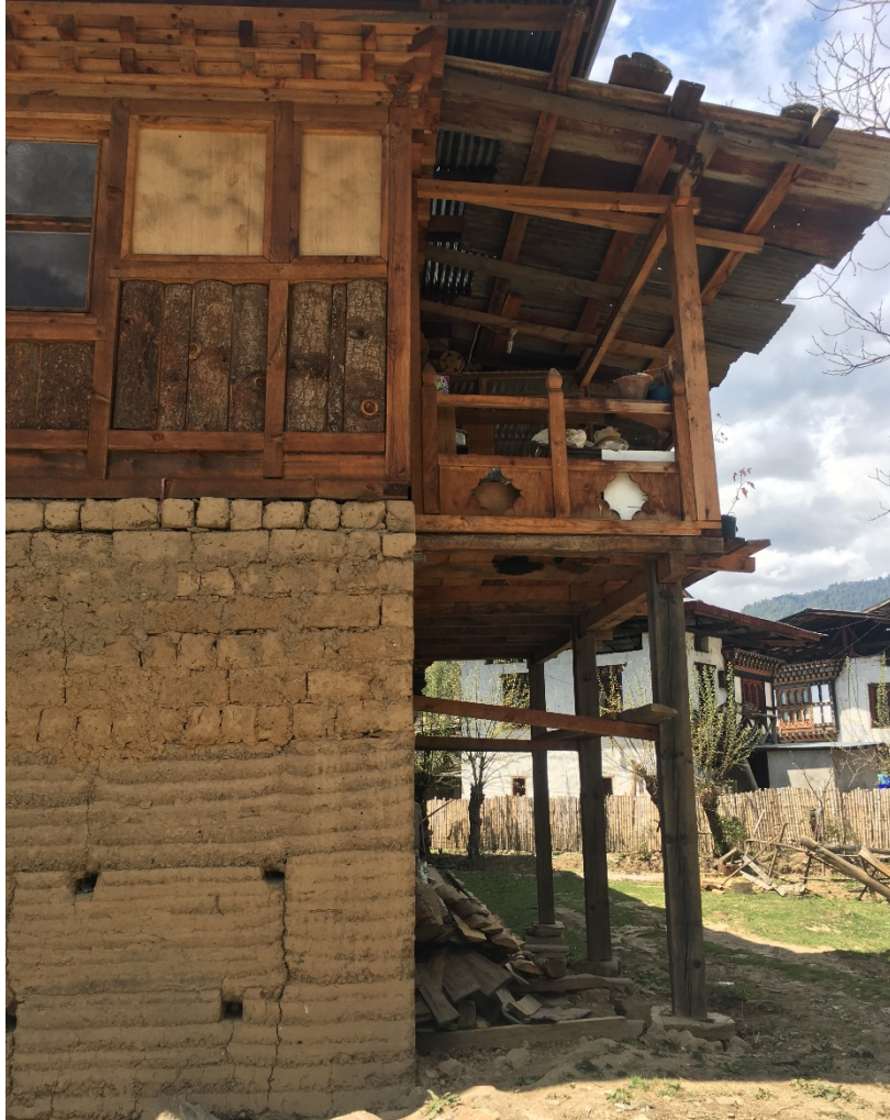
Figure 8: A Bhutanese building with a combination of earth building techniques
