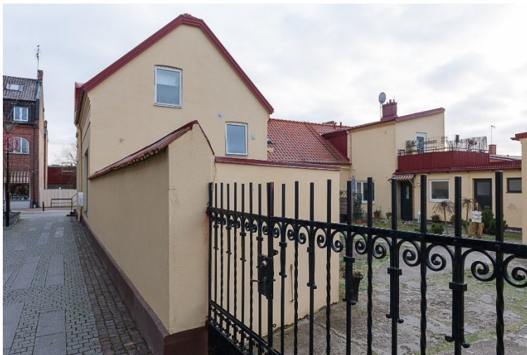
Figure 18 Yellow building on the corner of Stenhuggaregatan and Mårtensgatan
