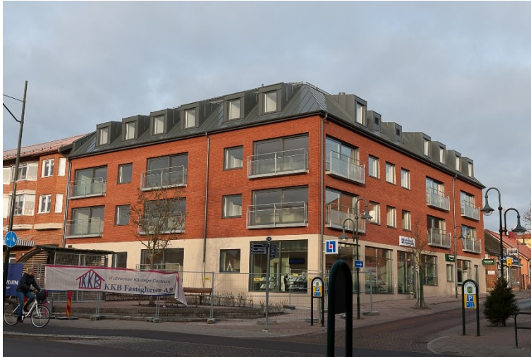
Figure 10 New building in traditional style, corner of Kvarngatan and Mårtensgatan
