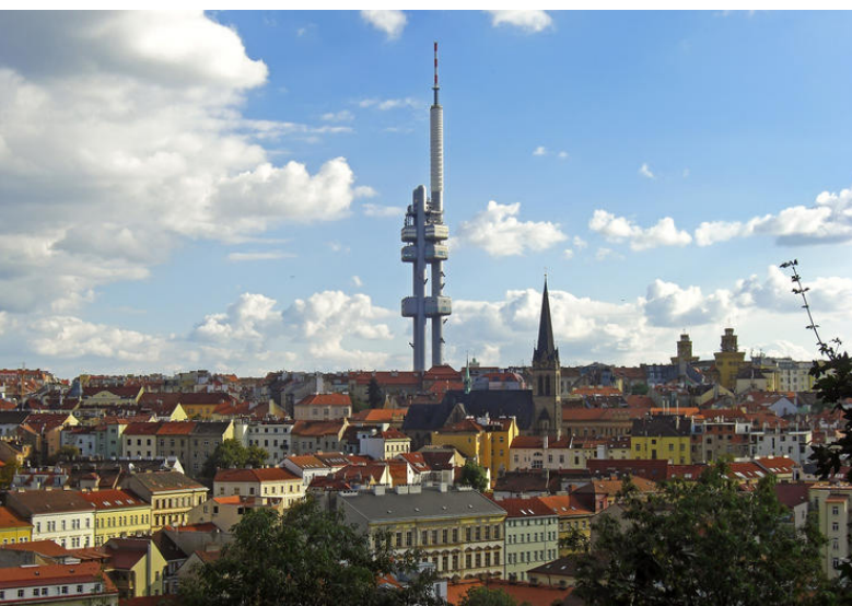
ŽIŽKOV TV TOWER, ROOFSCAPE
