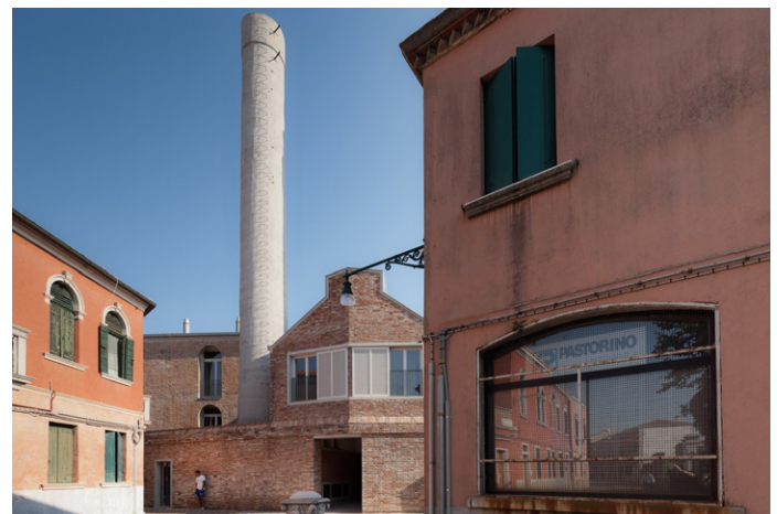
Two new residential complexes inside a disused factory SOURCE: https://images.adsttc.com/media/images/56dc/657a/e58e/cec3/ec00/0065/slideshow/portada_004.jpg?1457284467
