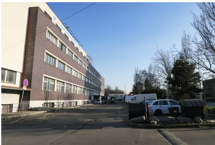
Front facade of the station Source: DS
