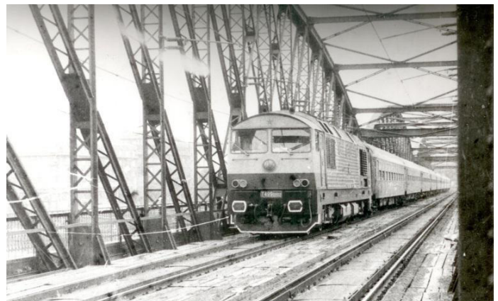
Railway bridge- connection to the right bank of the city
