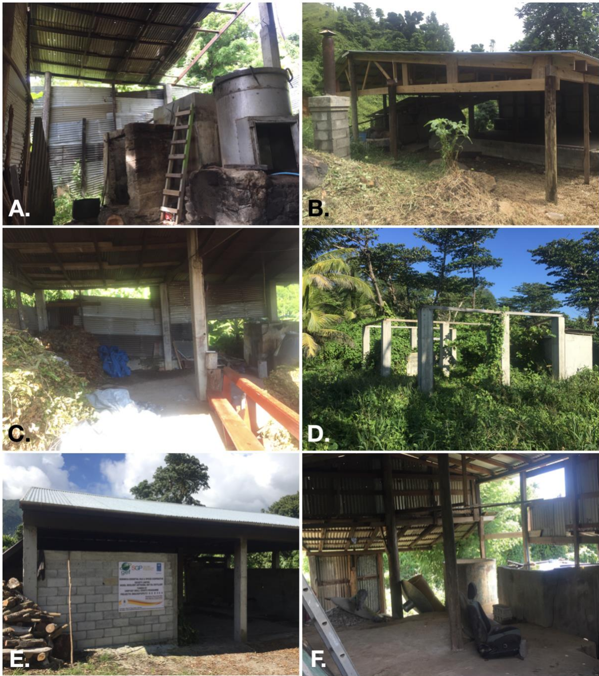
Figure 13: Some of the Distilleries visited and documented during field visits. A: the inside of a distillery under reconstruction. The owner recently took over his grandfather's distillery. Remotely located B: A newly rebuilt distillery, just a couple of months old, still not used at the time of the interview but easily accessible. C: A distillery rebuilt quite soon after Maria, quite easily accessible. The owner had several batches from other farmers waiting for distilling.. D: A damaged and abandoned distillery, however, only the roof missing. E: A recently reconstructed distillery sponsored by GEF Small Grants, it had electric lights and a washroom, also very easily accessible. F: A reconstructed distillery, the owner has installed zip-lines from close-by fields to facilitate transport of leaves, something many farmers talked about.
