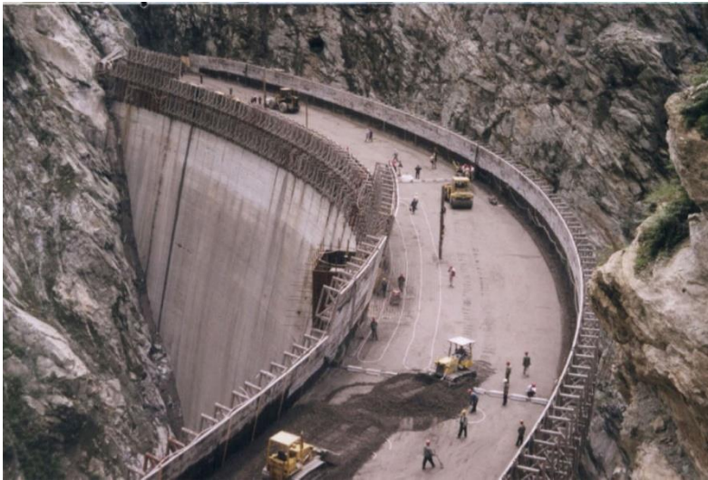
Figure 7. The Shapai dam during construction (Malcolm Dunstand and Associates, n.db)
