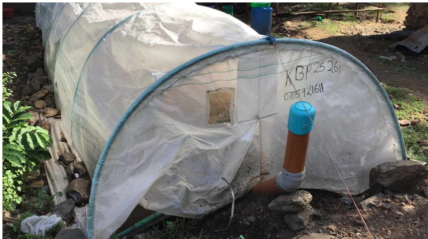
A MODEL OF THE DOMESTIC BIOGAS SYSTEM AT DUNGA BEACH. THIS MODEL COSTS $750 USD.
