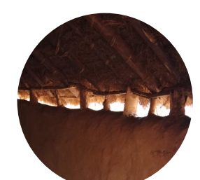
Light and ventilation gap between the roof and the ceiling
