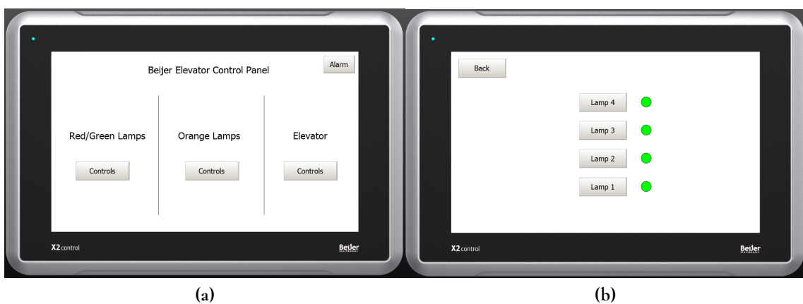
Figure 3.14: The interface on the Bejler display. (a) shows the home screen, (b) shows the view for controlling the red and green lamps.
