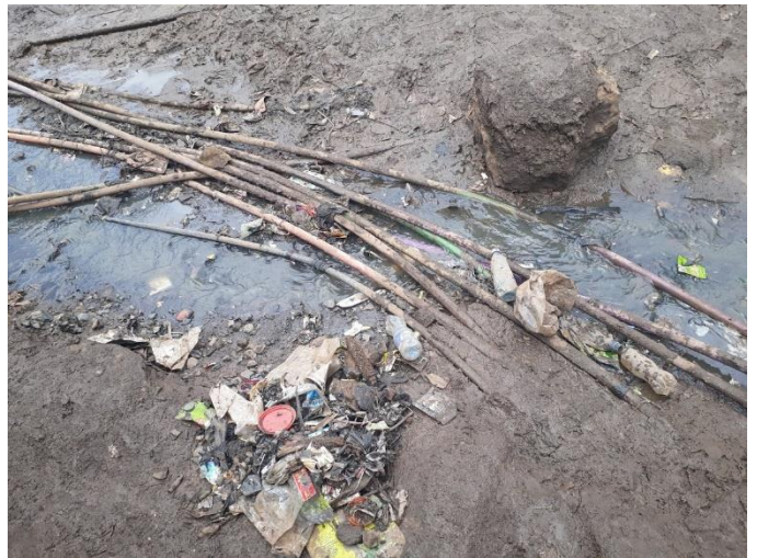
Image 2: Water pipes passing through sewage and waste
