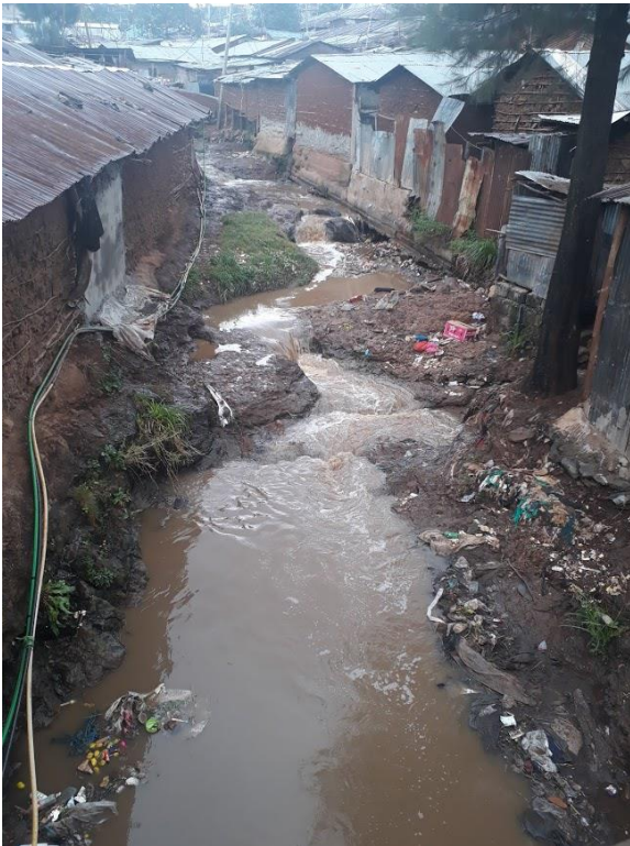
Image 1: Water pipes mounted to walls along the river
