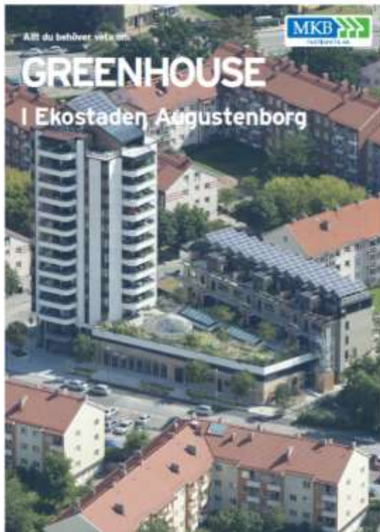
Fig. 5. Aerial View of the Greenhouse within Augustenborg Ecocity (Source: MKB Fastighets AB, 2018)
