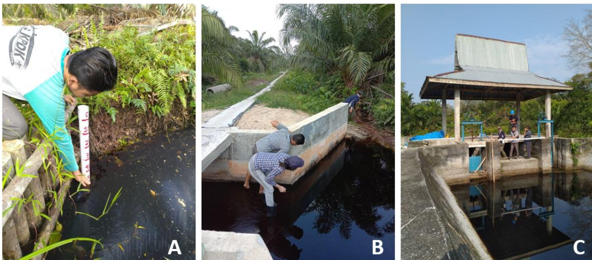
Figure 18 Canal Blocking, an intervention for fire prevention. a) small canal blocking in Group 3's plantation for monitoring the water contained in the peat soil by blocking the flow of water to keep the peat moisture. b) we were making a permanent measurement in the main canal to monitor the water level, and c) the main canal block. (Photos by the author and a local facilitator in Siak, January 26, 2020)
