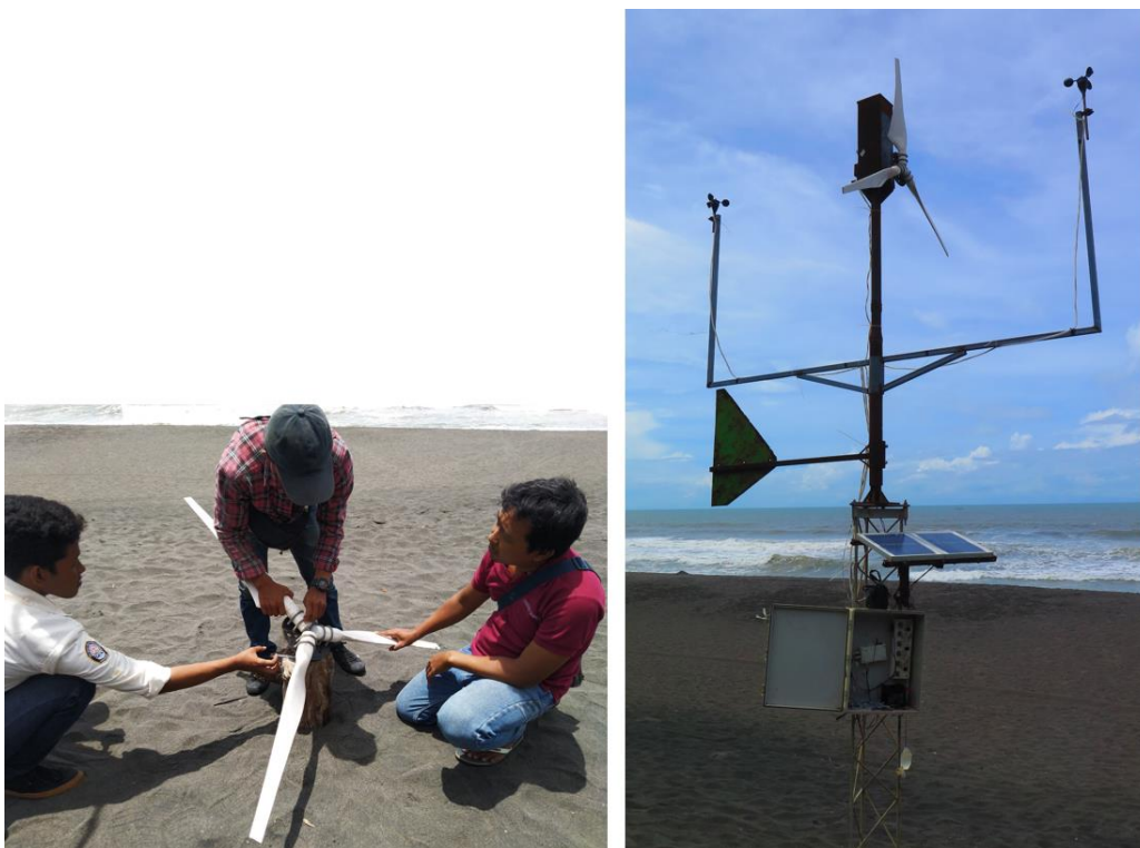
Figure 7. Daily activities of PLTH staff (2). A PLTH staff member with two students working on a wind turbine (left) to be placed in the wind turbine and solar panel combination tower (right) (Own photographs, 2020).
