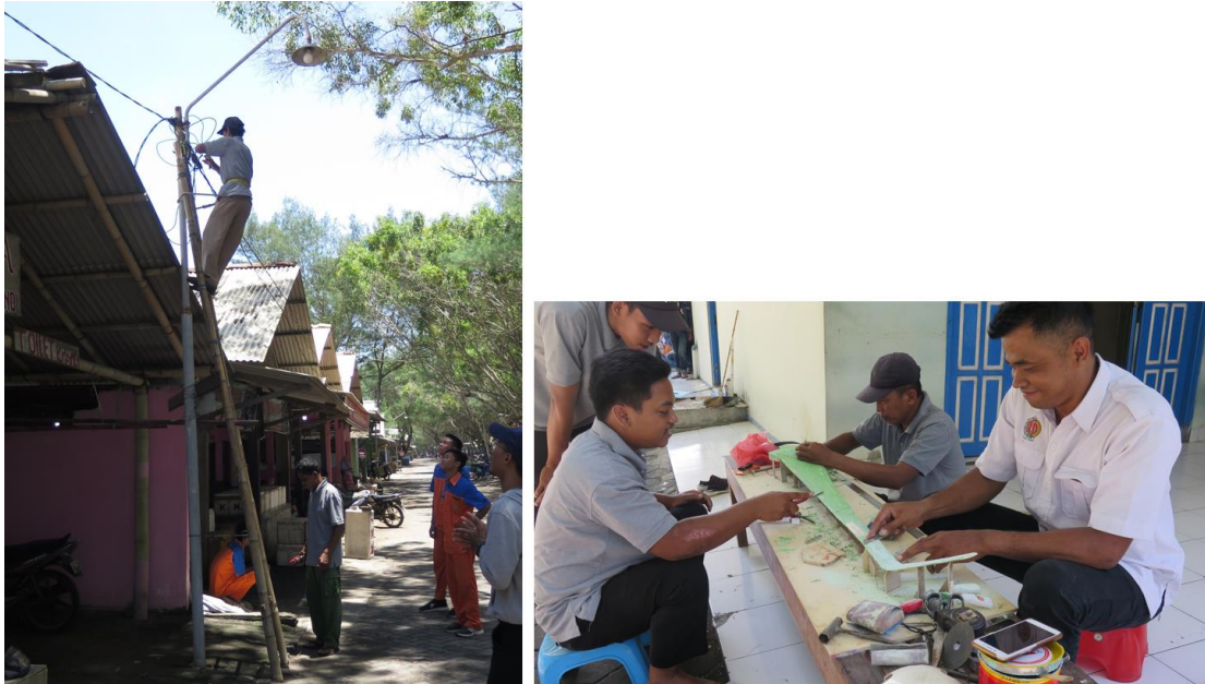
Figure 6. Daily activities of PLTH staff (1). Two PLTH staff was repairing cables for the streetlight while being observed by a group of students (left), and some PLTH staff were building a wind turbine (right) (Own photograph, 2020)
