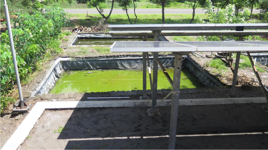
Figure 4. Freshwater fishponds below solar panels on a sandy soil built by the project initiators and oxygenated with PLTH electricity (Own photograph, 2020).
