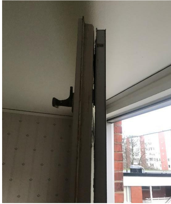
Figure 4 The window of the existing building
