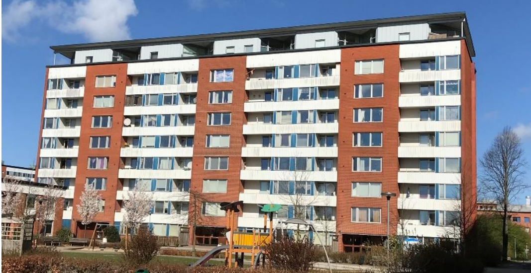
Figure 5 The façade of the building A1
