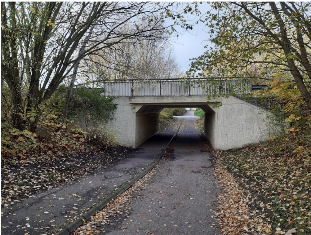
Figure 38. Example photo of tunnel with crossing bicycle road afterwards. (2019-11-07).
