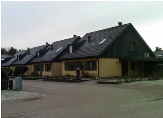
Figure 2. Typical single-family buildings built during the million program. Photo by Karlstad Kommun (karlstad.se)
