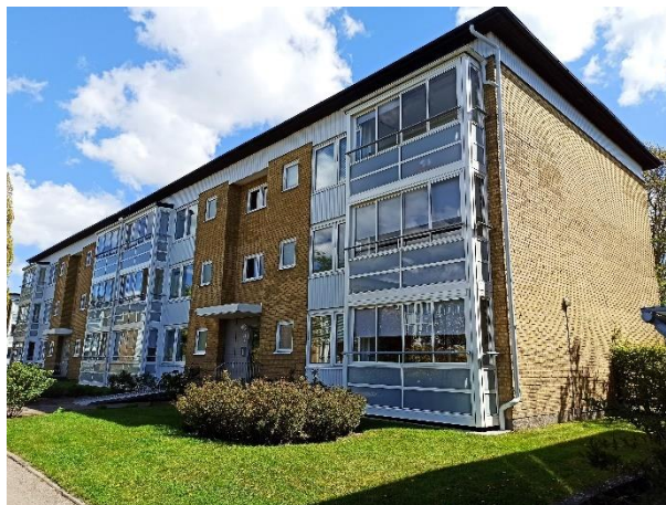
Figure 1. Typical three story multi-family building built during the million program. (Photo by authors)
