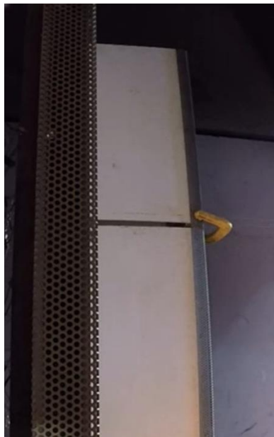
A11. c) Live Fire Test Perforated Cavity Lateral Obstruction
