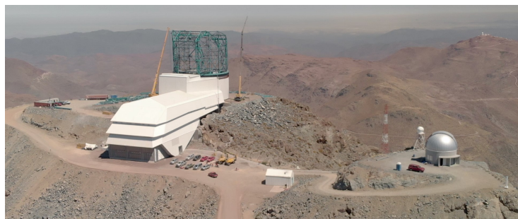
Figure 4: LSST under construction in summer 2019 ( LSST, Telescope & Site ).
