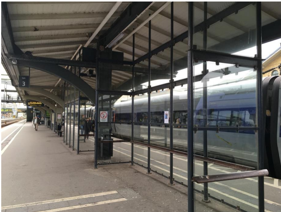
Figure 11. Glass shields at Lund Central Station
