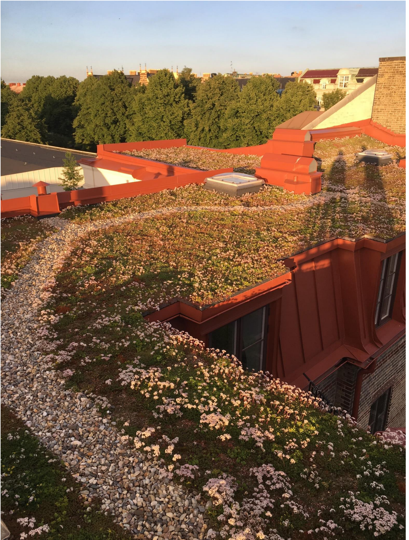
Credit: Peter Arnfalk – extensive green roof in Malmö, Sweden
