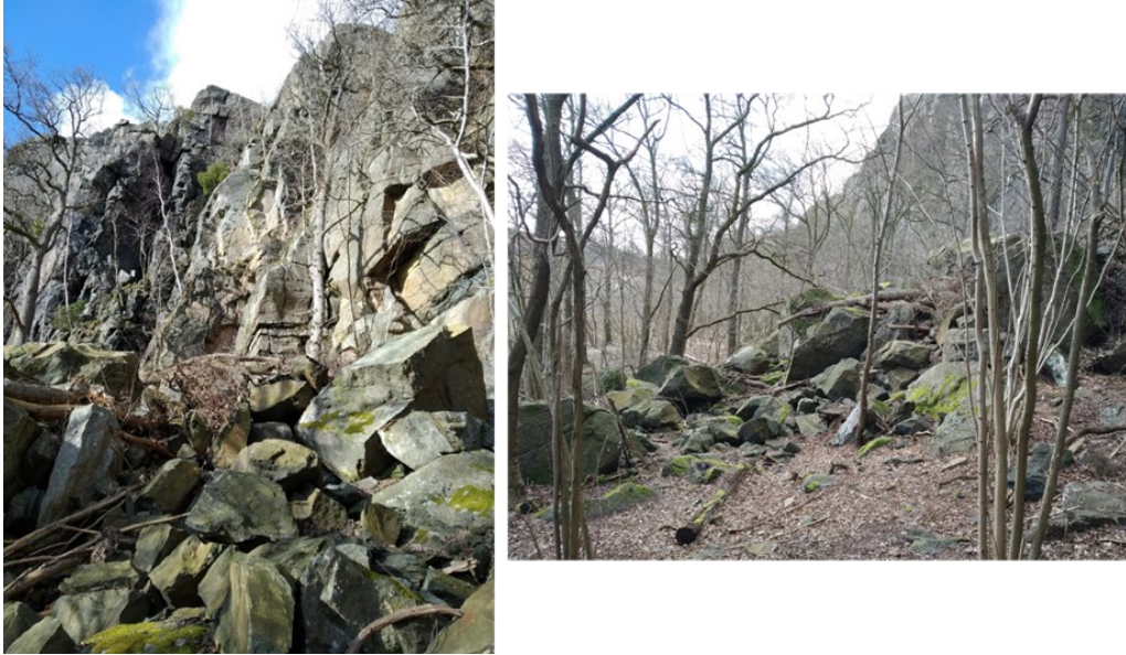
Fig. 26. The 2017 rockfall. Front view to the left, lateral view to the right. To see details of the extent of the rockfall, see Section 5.4.
