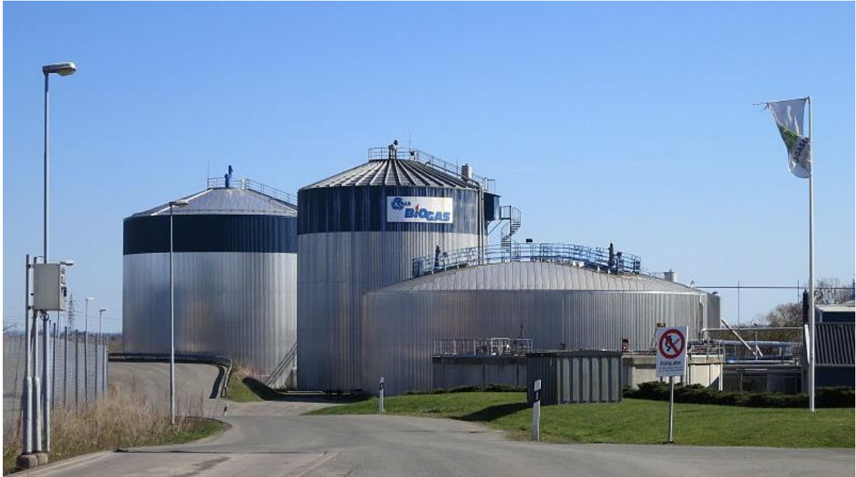
Figure 1. Karpalund biogas plant. Image downloaded from Wikipedia: Biogasanläggningen Karpalund https://sv.m.wikipedia.org/wiki/Karpalund .
