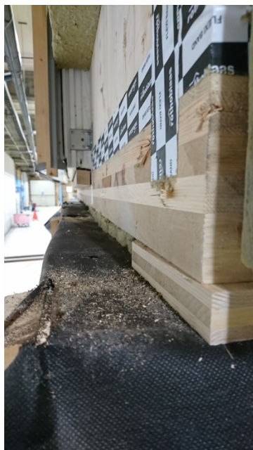
Figure 26 - Wooden blocks intermediate layer
