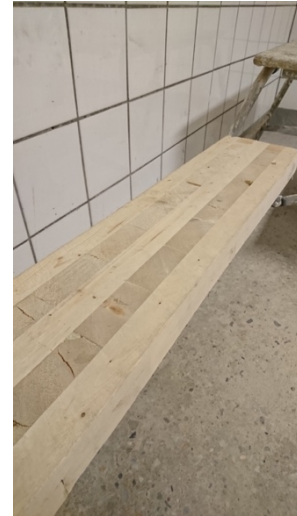
Figure 4 - CLT-floor cross section
