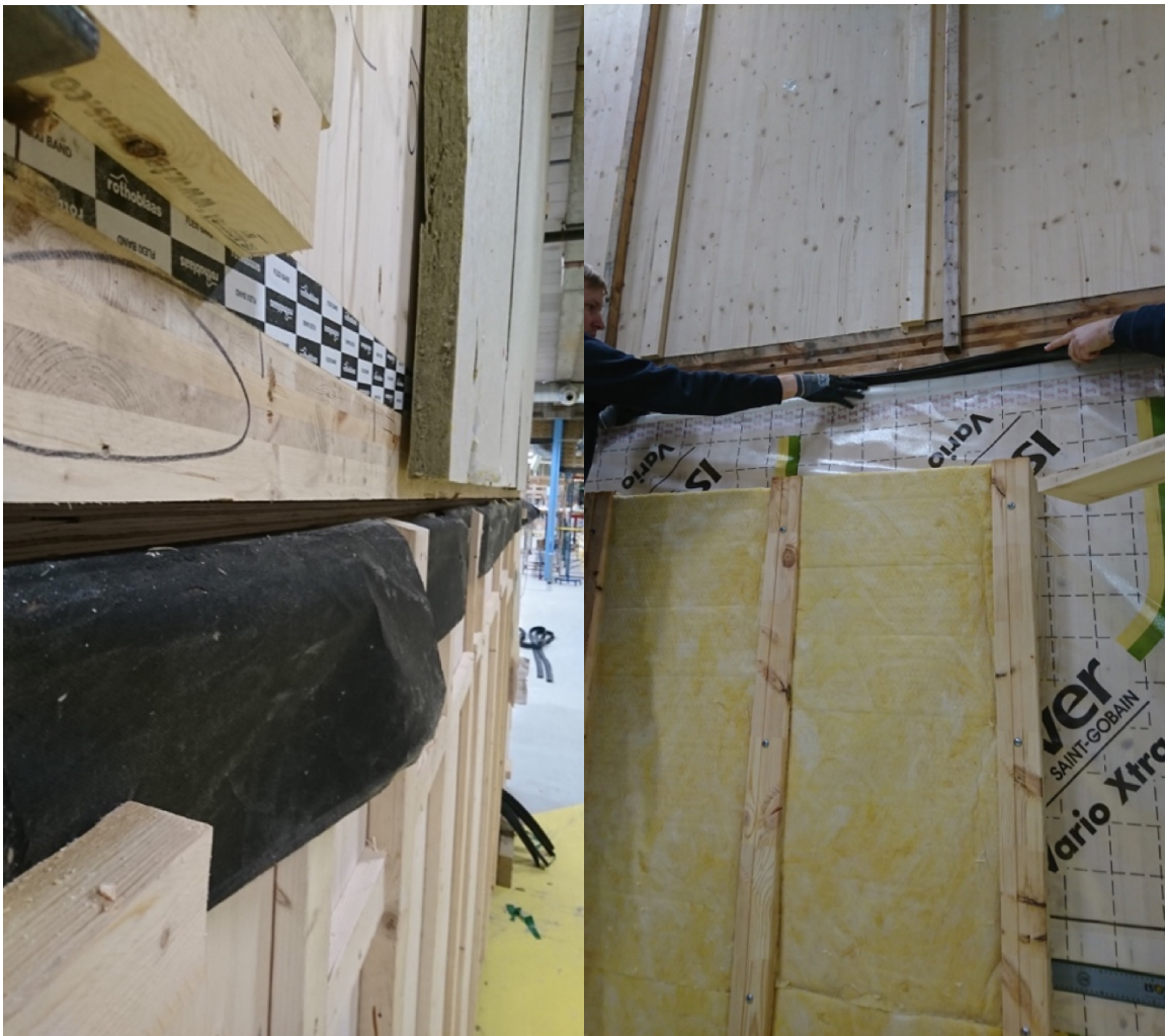
Annex E: Intermediate Layer, factory conditions
