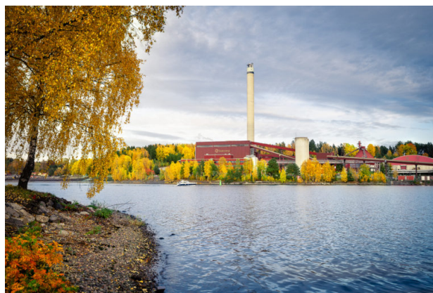
Figure 1.1 The Ingelsta CHP located in Södertälje, south of Stockholm [6].
