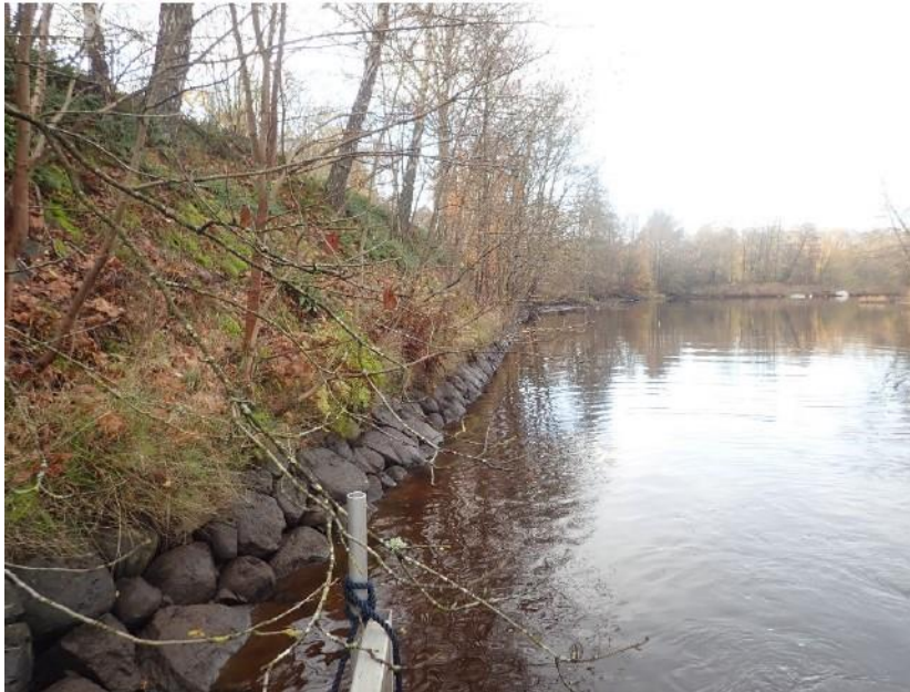
Figure 4.4: A typical river section showing various roughness condition in the overbanks (Grännsjö, 2020)
