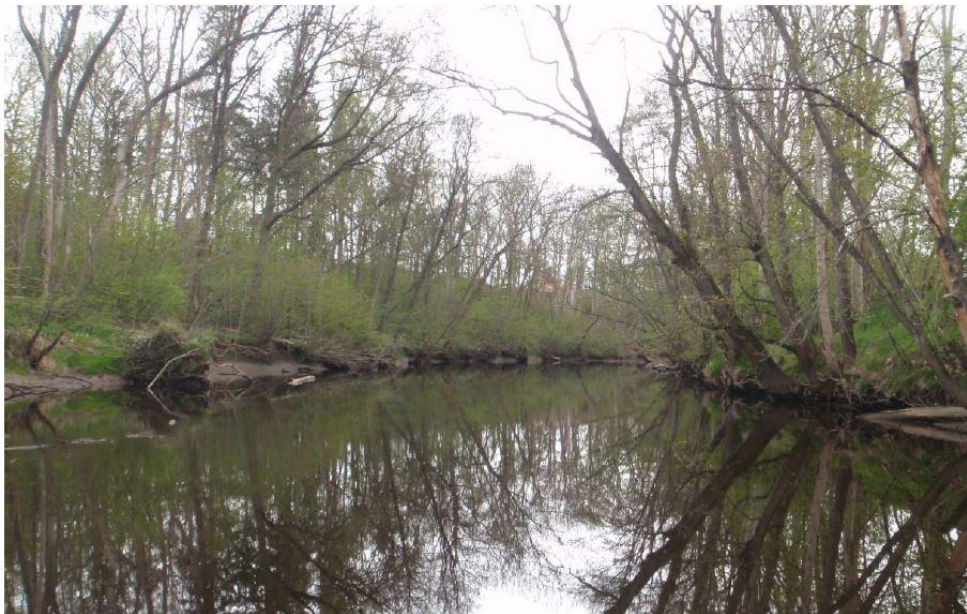
Figure 4.5: An example of typical erosion problems at Ängelholm causing trees to fall into the river (Almström, 2010).
